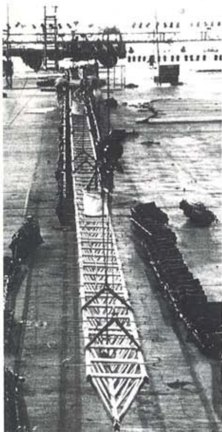
"The longest truss in the world" - for the 1987 Royal Tournament at Earls Court. The event is an annual four-in-hand between producer Major Michael Parker, lighting designer Robert Orno, Theatre Projects and The Unusual Rigging Company Limited.
