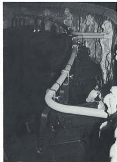
Lighting bars fixed to tier fronts are easily removable - the auditorium can be returned to a totally 'clean' state with a minimum of fuss.
