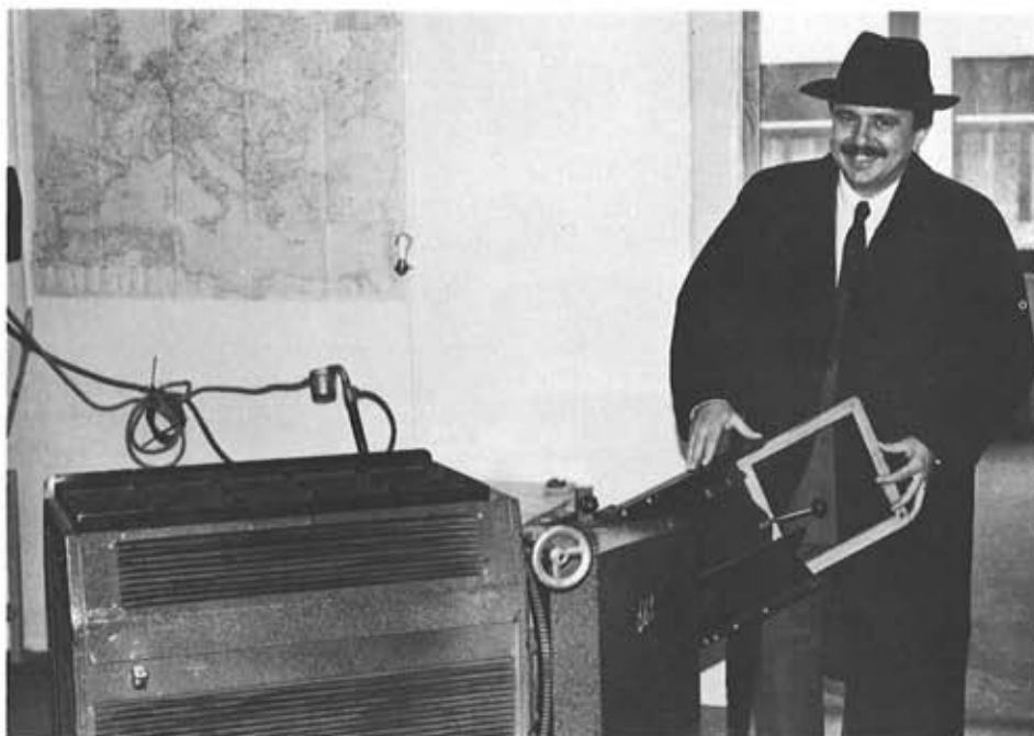
Hermann Sorger pictured with a BP10 10k scenic projector in for service from the Vienna Staatsoper. This unit was specially designed for bridge work, with a special front end mirror system.
