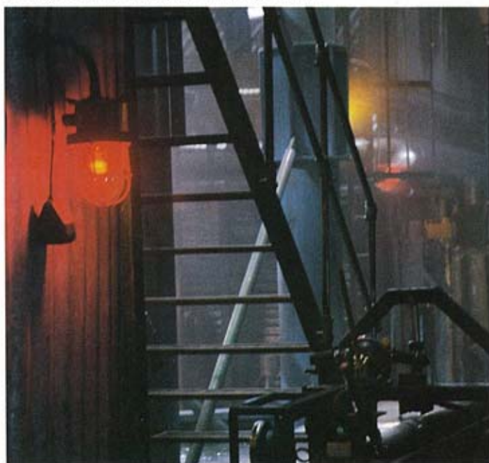
A red bulkhead and a coolie shade with 40W incandescent give that authentic industrial feel.
