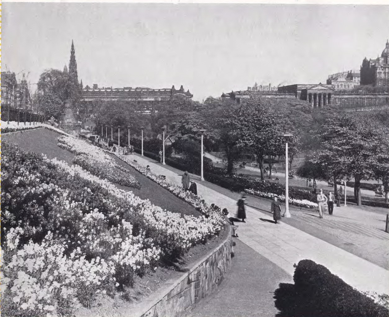
Edinburgh. Princes Street Gardens. Mushroom lanterns on concrete columns.
