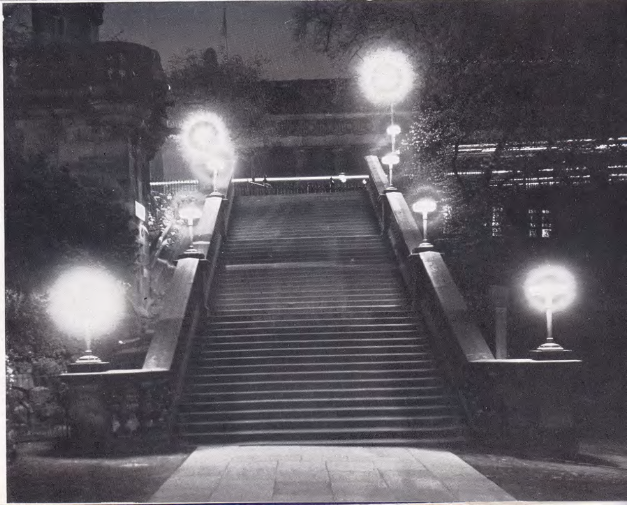
Night view of steps lighted by the type of pedestal-mount- ed balustrade lantern shown above.
