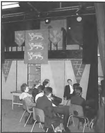
▲ Queen Elizabeth's School, Mansfield, Notts. Mid-19th century class room converted to a video studio with the aid of drapes, lighting grid, luminaires, Tempus control and dimmer packs supplied and installed by Strand.
