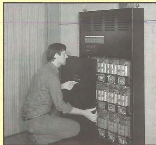
Permus Dimmer Rack
