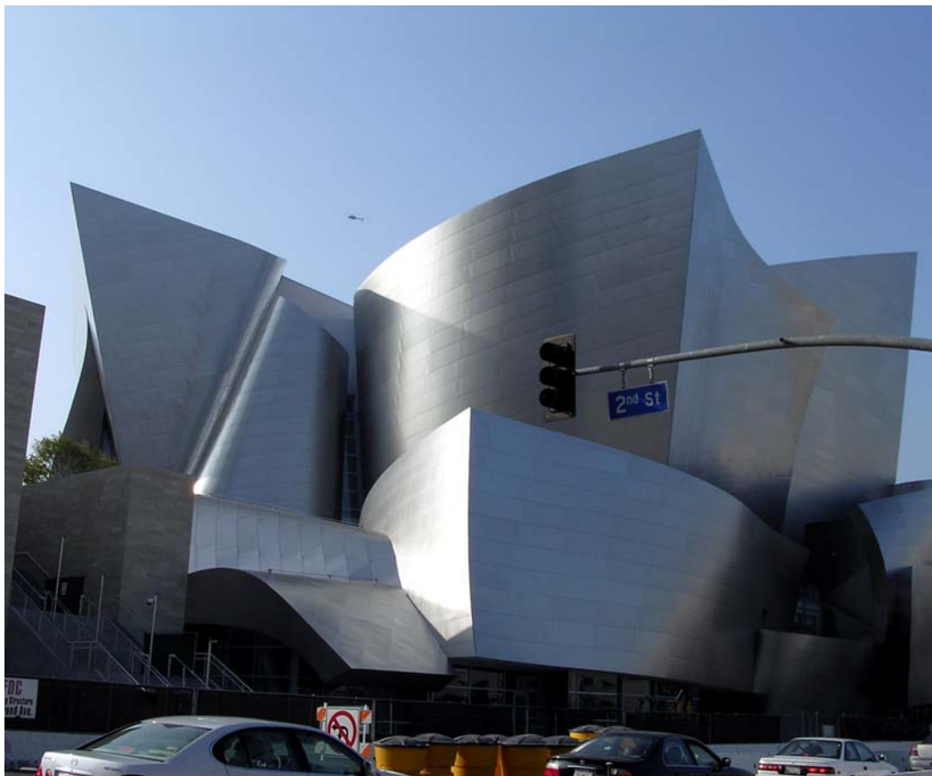
A view of the theatre from Grand Avenue. Photo Courtesy Theatre Projects
